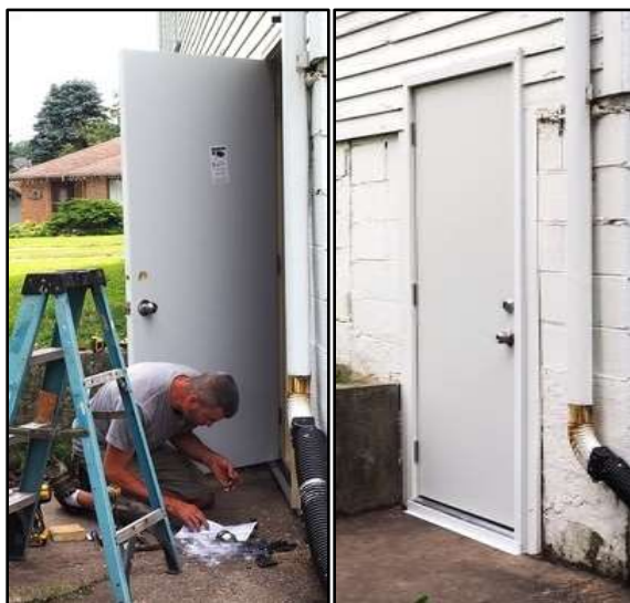
Seaton Replaces the Museum's Northeast Door
