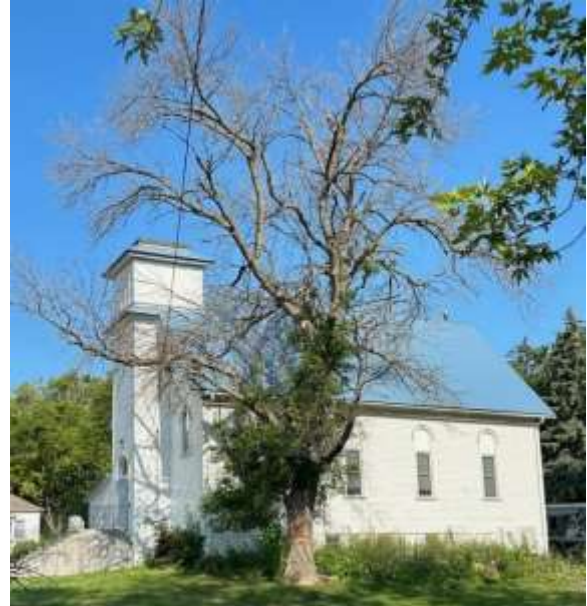
Tree Removal Begins
