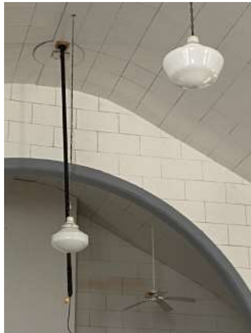
Old light fixtures
