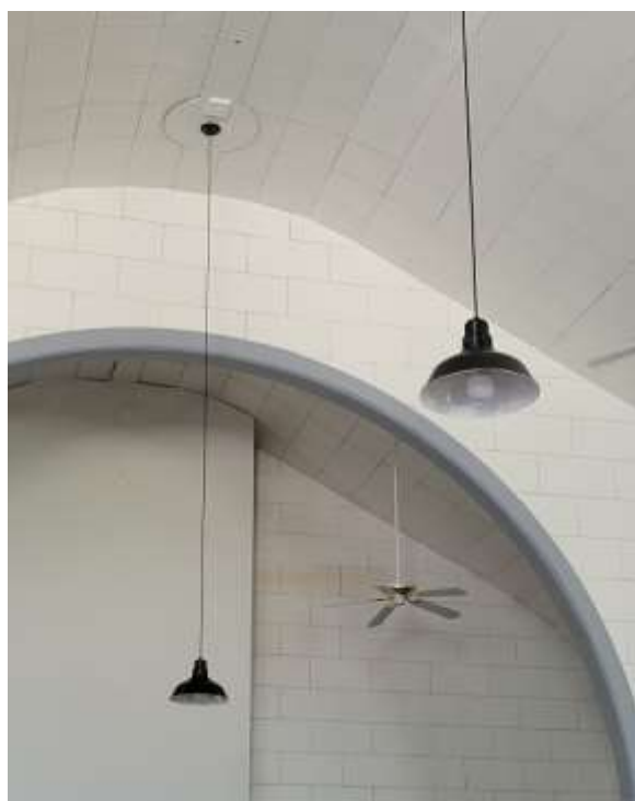
New Light Fixtures
