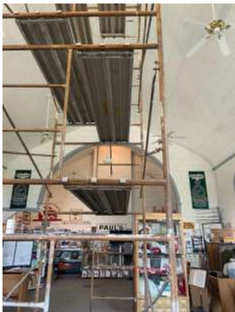
Light fixture replacement begins
