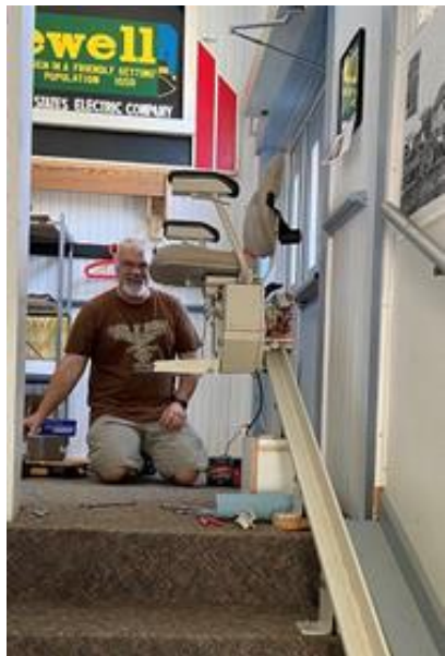
Contractor Ron Cook completes the installation
