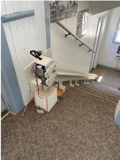
Lift mechanism installed
