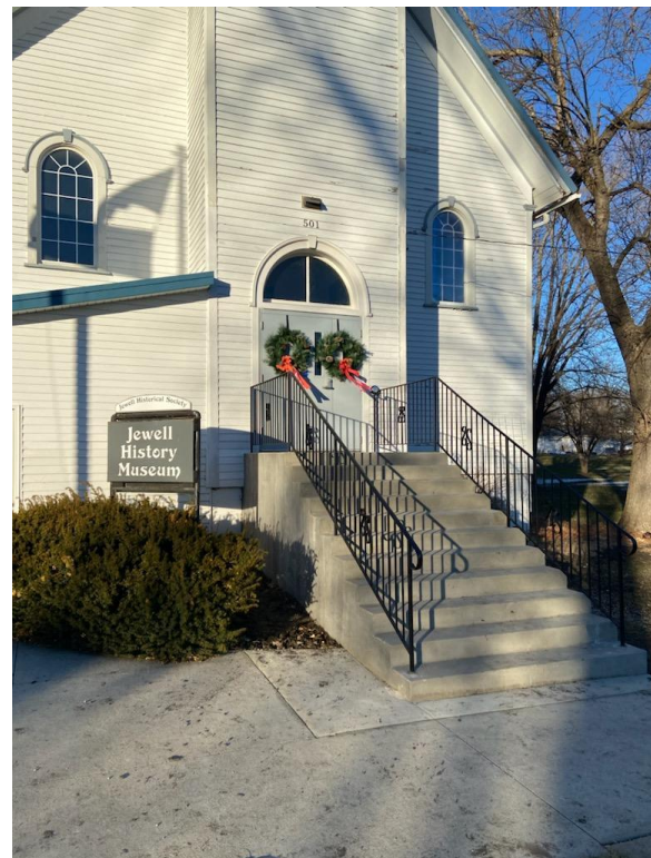
The completed front entryway.
