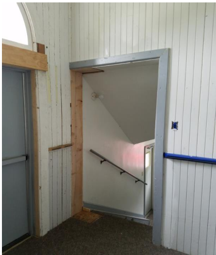
Interior stairway where chairlift will be located.
